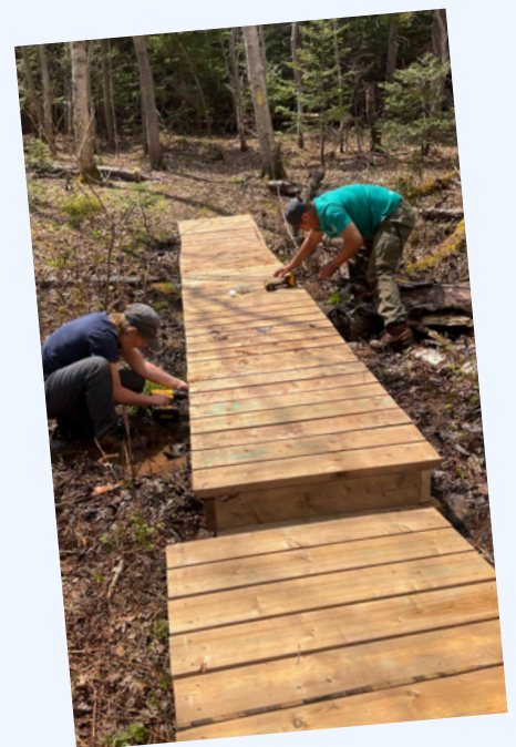
A boardwalk was installed at the Kildare Forest Natural Area to reduce trail degradation in wet areas. This was made possible by the PEI Active Transportation Fund.
